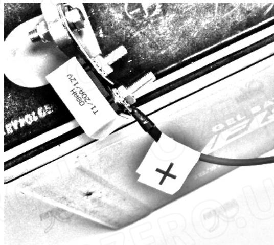
Using a product without a thermal relay can lead to a fire and a threat to your life! By no means change its position and disconnect it from the power cable!
